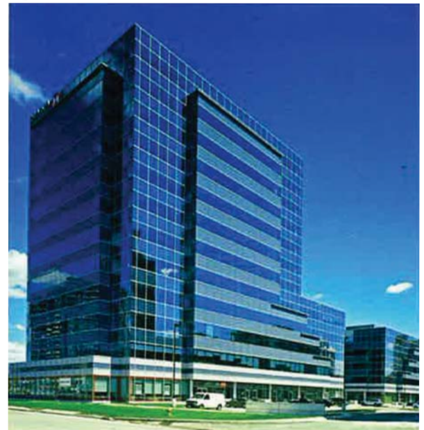
Liberty Square buildings on Highway 7 across from the Markham Civic Centre.
